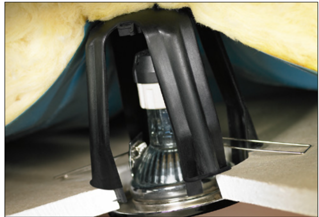
SpotClip-II ensures reliability and safety of lighting installations.
