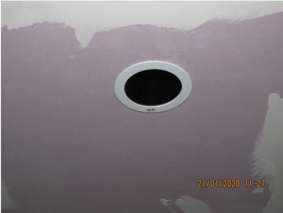
Frame 1: Downlight 1 exposed face pre-test
