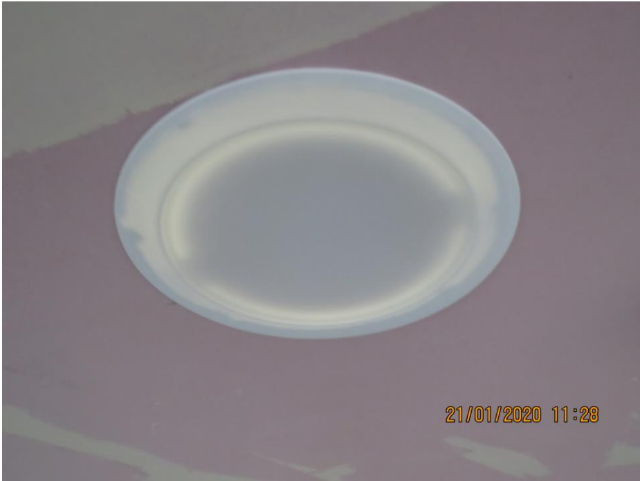
Frame 7: Downlight 3 exposed face pre-test
