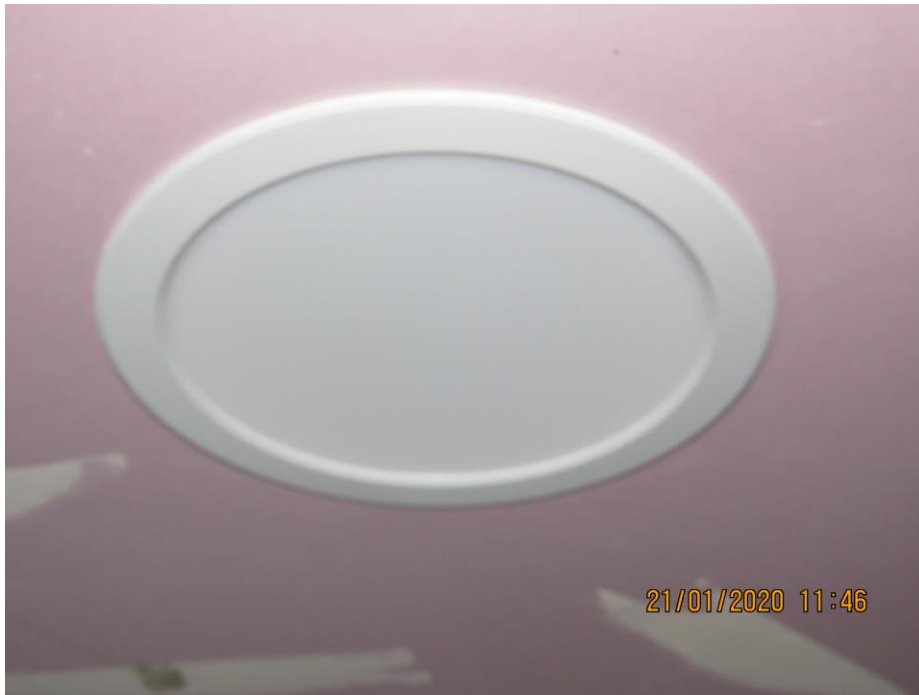
Frame 19: Downlight 7 exposed face pre-test
