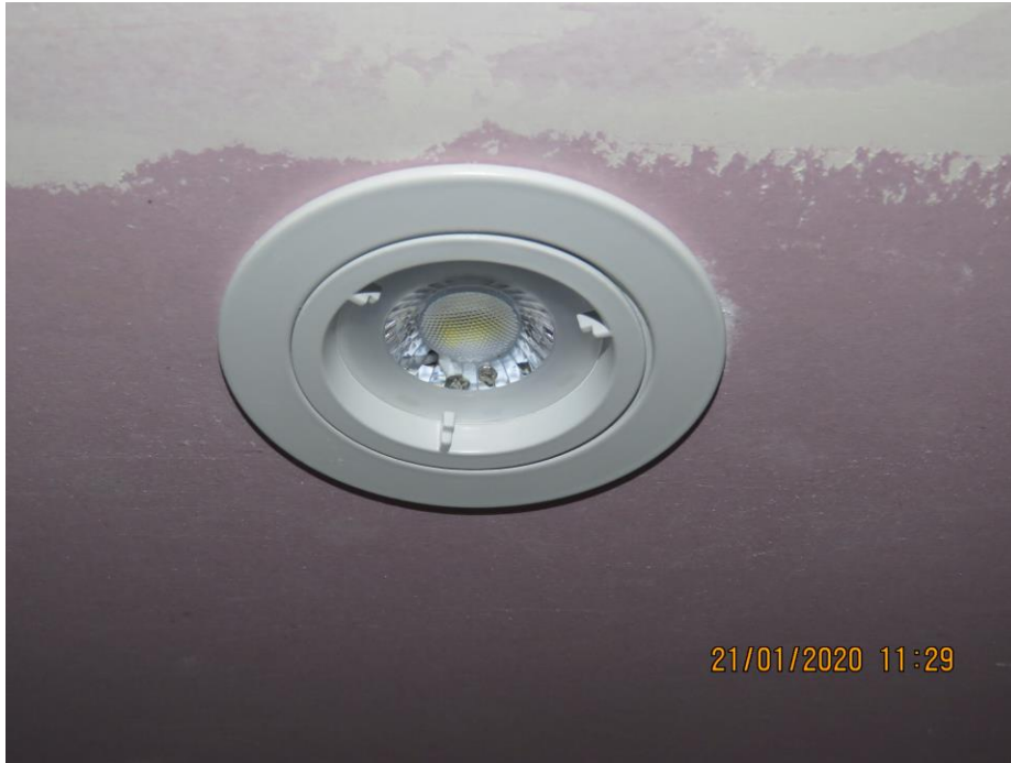
Frame 13: Downlight 5 exposed face pre-test
